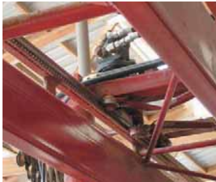
Log's-eye view of the overhead track. The feed mechanism is a hydraulic motor with a gear that engages in a chain welded to the side of the track.
