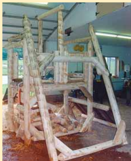
Some joints and splices require special fastening, in some cases a timber lock lag driven in with impact drive.
